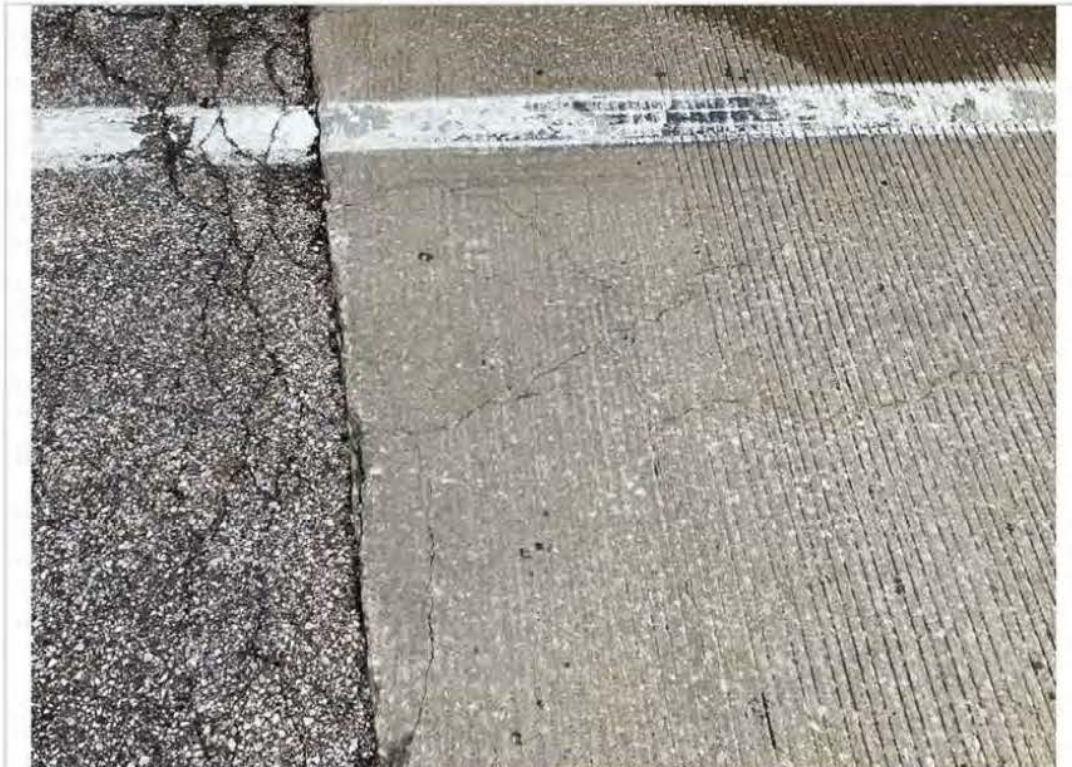
Span 3 cracks
