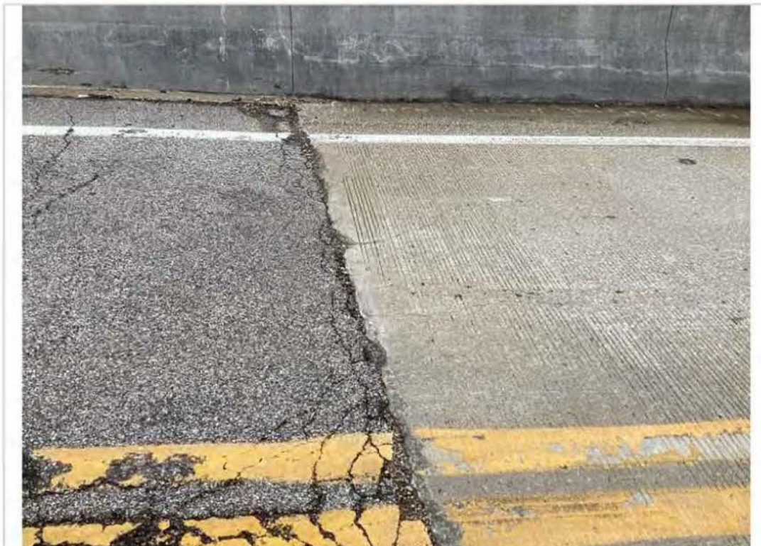
Span 1 spall
