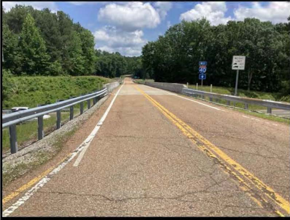
Approach 1 weight limit sign @ 26.47 bridge
