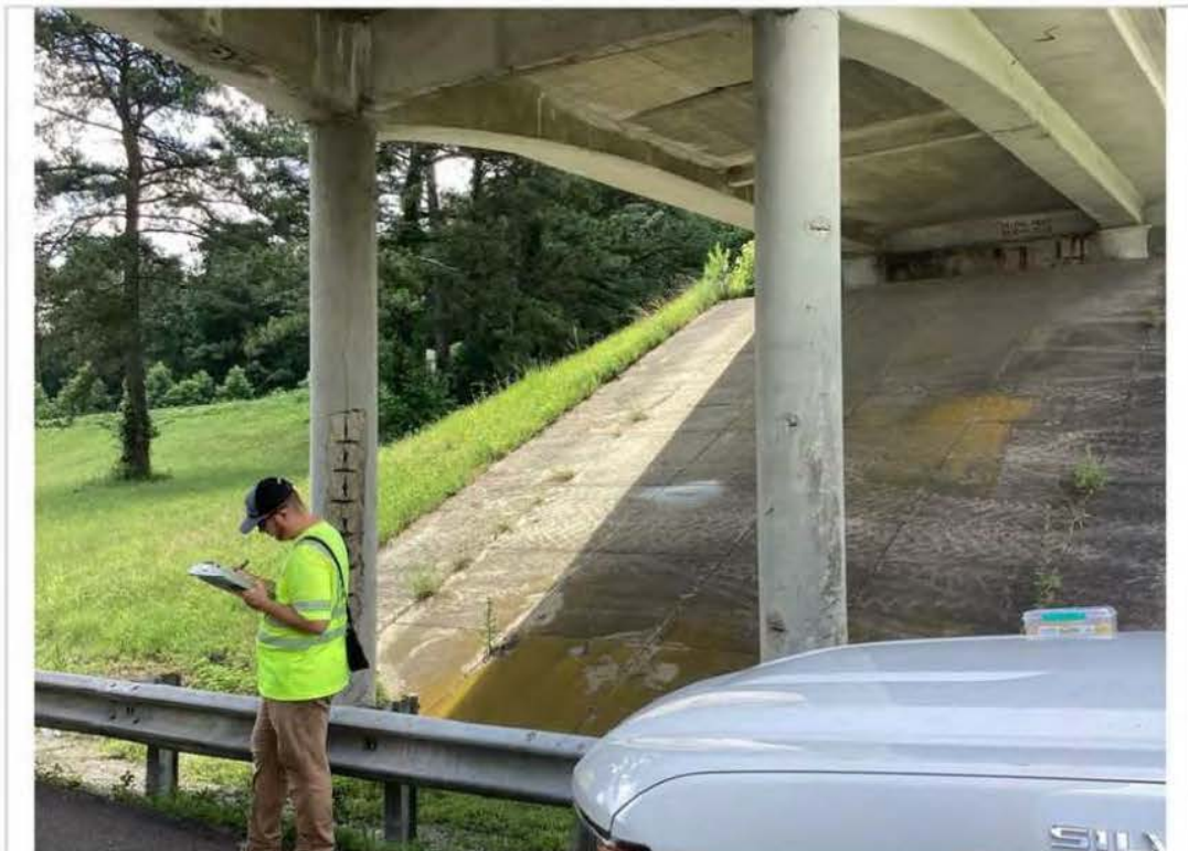
Bent #1 looking back
