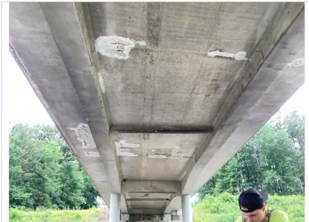
Bottom deck of span #2
