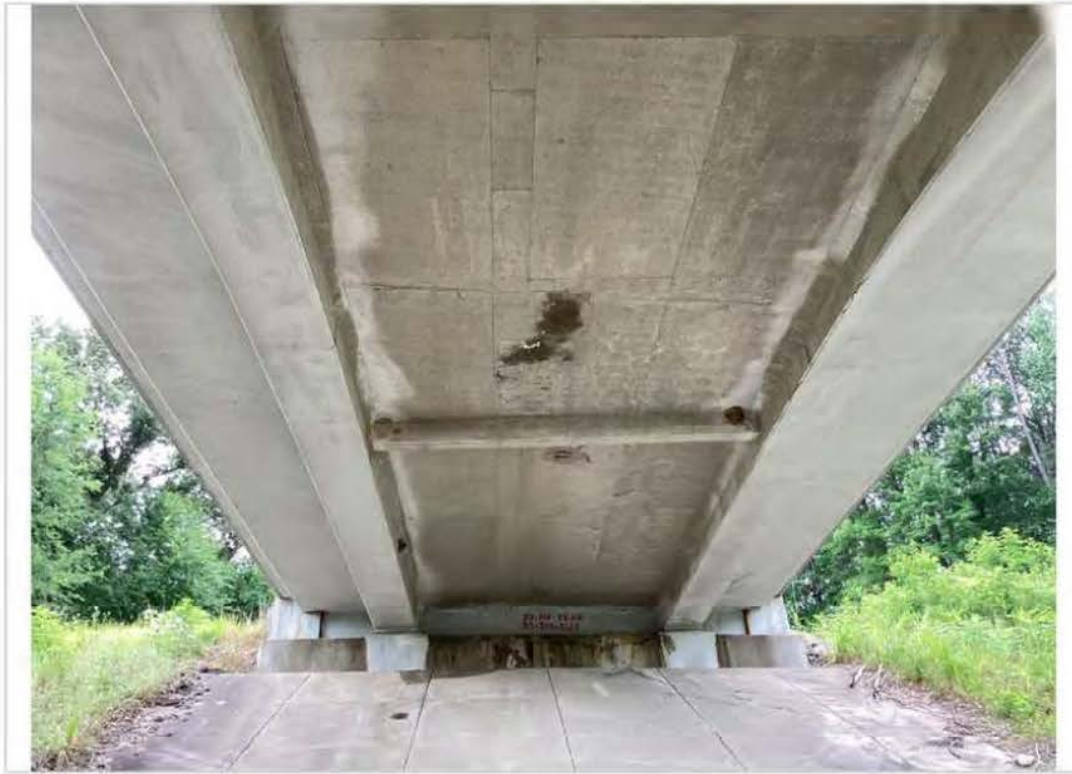
Span 1 bottom deck typical
