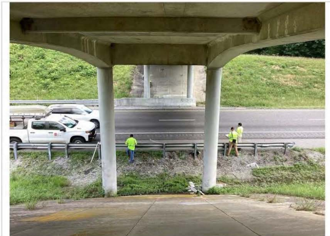
Bent #1 looking forward
