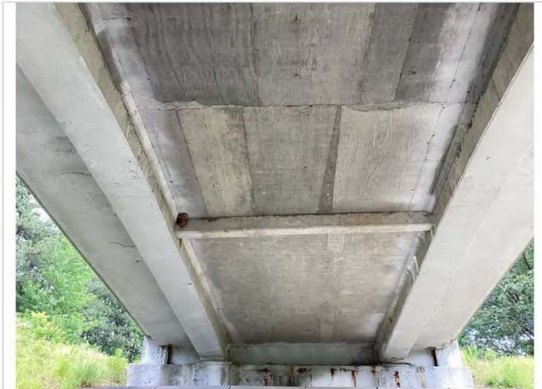
Bottom deck of span #3
