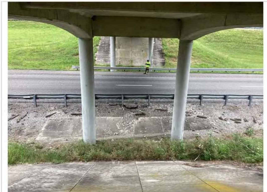
Bent #1 looking forward
