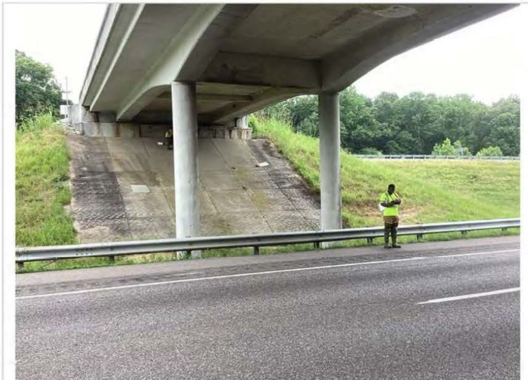
Bent #2 looking forward
